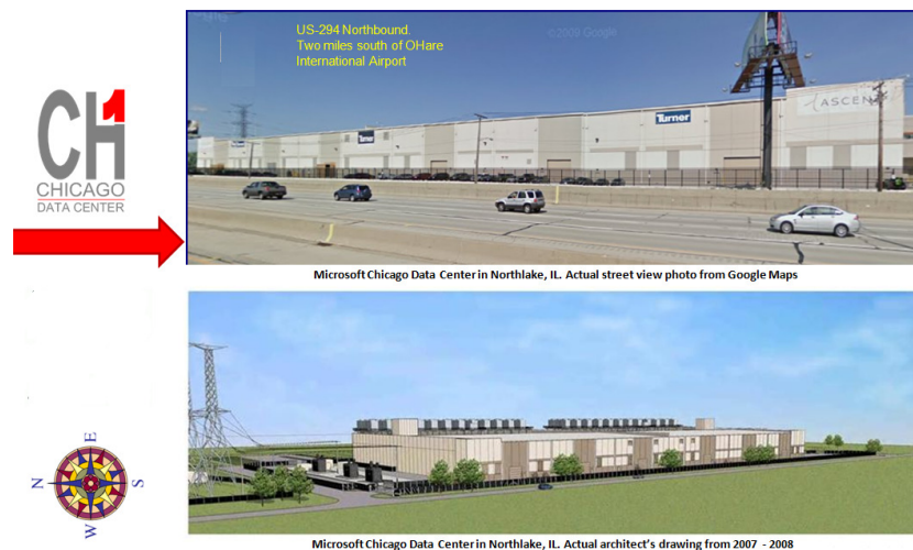
Figure 1 – Side Views of the Microsoft Chicago Data Center
