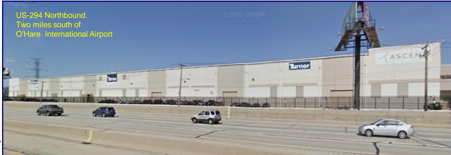
Microsoft Chicago Data Center in Northlake, IL. Actual street view photo from Google Maps
